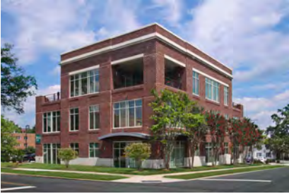
Bragg Building 1031 South Caldwell Street, Charlotte
