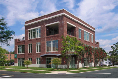
Bragg Building 1031 South Caldwell Street, Charlotte
