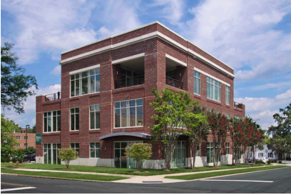
Bragg Building 1031 South Caldwell Street, Charlotte
