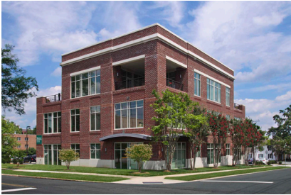
Bragg Building 1031 South Caldwell Street, Charlotte
