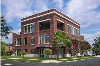
Bragg Building 1031 South Caldwell Street, Charlotte
