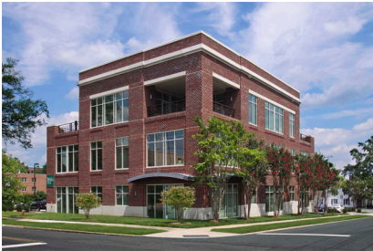
Bragg Building 1031 South Caldwell Street, Charlotte
