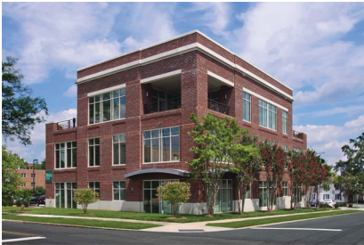
Bragg Building 1031 South Caldwell Street, Charlotte
