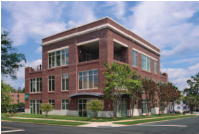
Bragg Building 1031 South Caldwell Street, Charlotte
